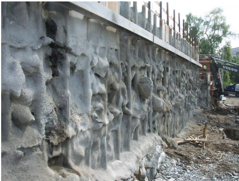
Fig 14. Shotcrete used to fill gaps between drilled tubes.
