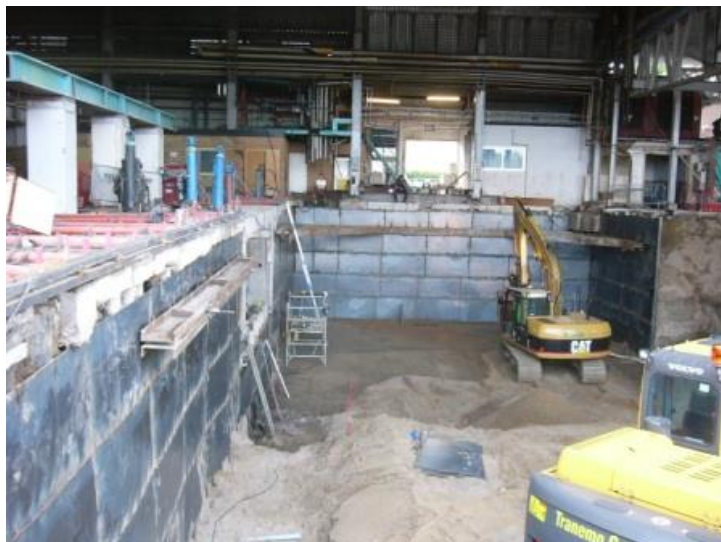
Figure 9. Drilled Micro Pile wall for the Rexam glass industry in Limmared, 2007
