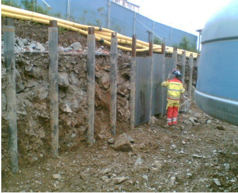
Fig 13 Excavation between drilled tubes
