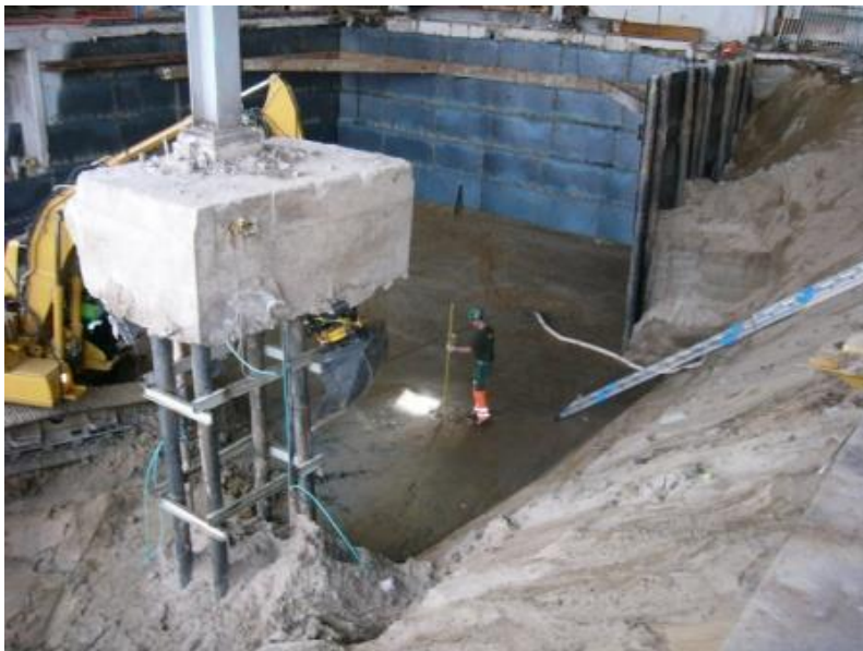
Figure 11 Drilled micro piles for temporary support of columns
